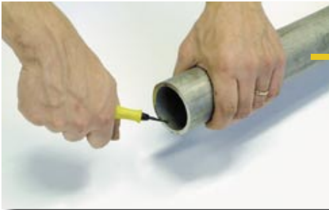
The pipe is first deburred inside and out; and cleaned...
